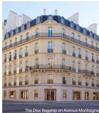
The Dior flagship on Avenue Montaigne.
