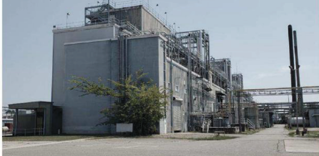
The Syre "blueprint" plant in Cedar Creek, N.C.
